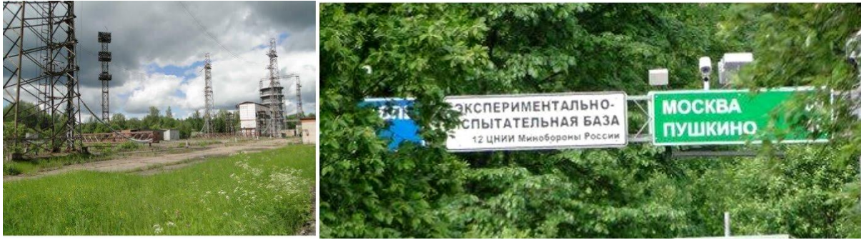
Fig.1.51c. Experimental and testing facility of CR&DI-12 (Moscow region)
