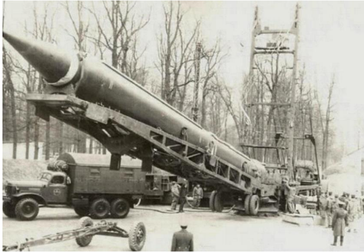
Fig. 1.47. Placement of R-12 missile (SS-4 Sandal) on a launching cradle
